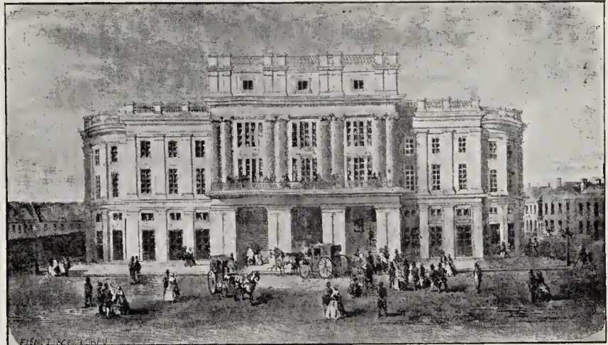
585 The French Opera House of New Orleans, built in 1821, from a French print, 1856, in the New York Public Library
